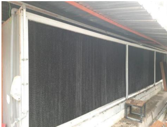
Gambar 33. Perbaikan cooling pad Closed House Japfa
