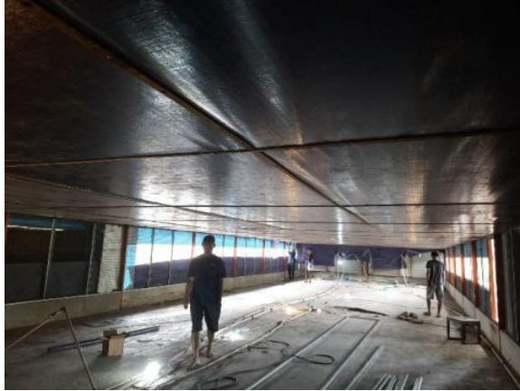
Gambar 32. Renovasi kandang Closed House Japfa
